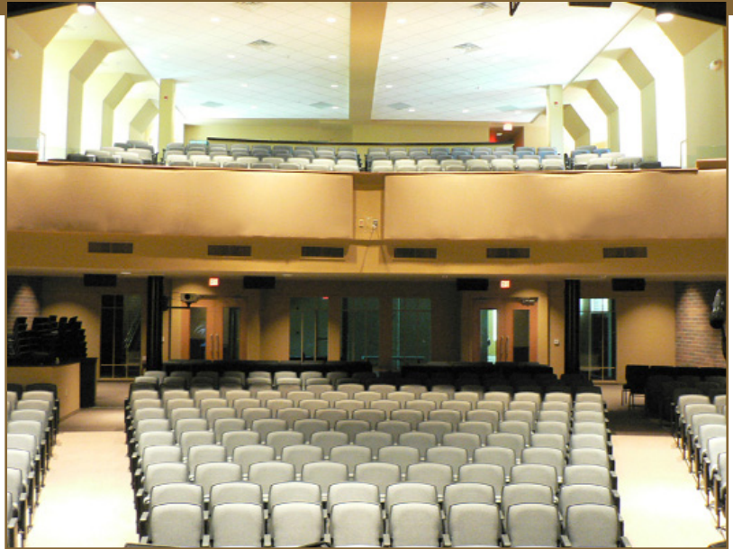
The choir and director at the new life church were getting a significant echo caused by the curved flat surface that made up the structure of the balcony. Because the building was brand new, they needed a decorative acoustical panel that would fit the curve of the large, flat reflective area.
