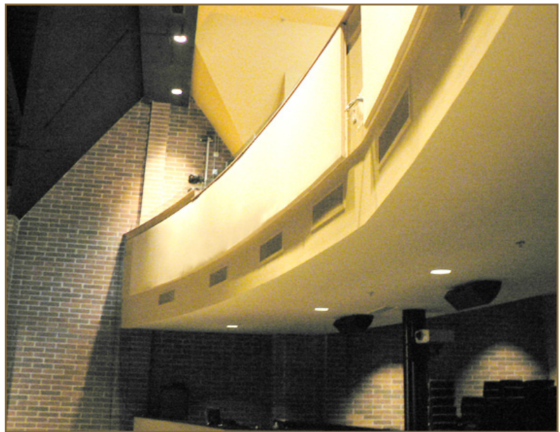
Because the building was so new, this customer did not want to adhere the cotton panels to the wall before they stretched the fabric – which is STRONGLY recommended. The concern was that they did not want to do anything that would have such a “permanent” affect on the room. After the fabric was stretched, it began to sag slightly, taking away the sharp borders of the track.
