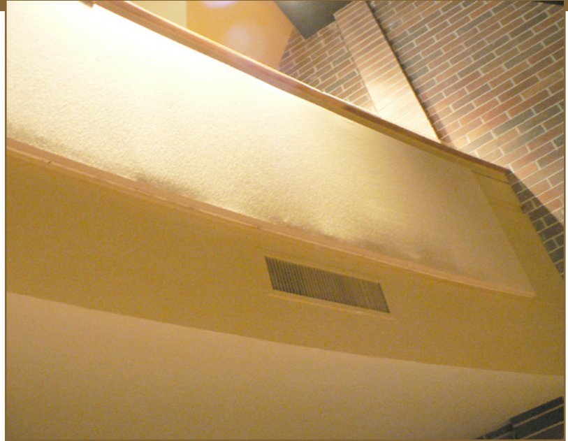
Because the building was so new, this customer did not want to adhere the cotton panels to the wall before they stretched the fabric – which is STRONGLY recommended. The concern was that they did not want to do anything that would have such a “permanent” affect on the room. After the fabric was stretched, it began to sag slightly, taking away the sharp borders of the track.
