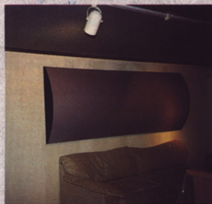
Photo 11: Rear wall parabolic reflector minimizes short reflections in the room.
