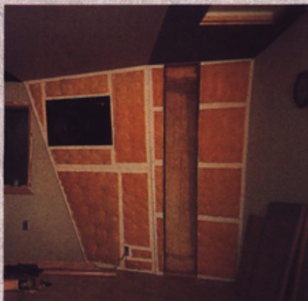
Photo 10: Laying insulation to absorb energy at the front of the room.
