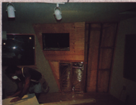
Photo 9: Enclosing the corner resonator areas.
