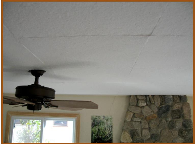
*In this installation, 1" thick, #3 lb. density Echo Eliminator panels in white were used. We cut these panels as straight as possible. With installations like the one pictured here, one can expect a certain amount of "quilting" or visible edges of the panels. Overall, the Echo Eliminator panels were used in this case because of the pure white color, as well as the cost effectiveness of the product.*
