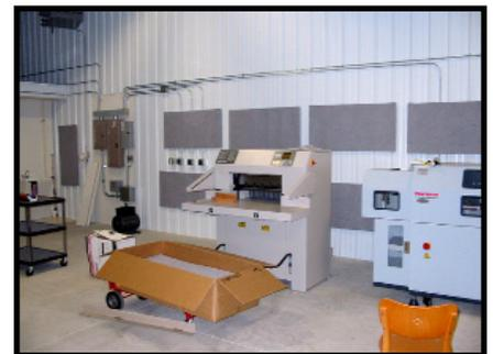
*Based on the cubic volume of this room, fifty-six panels were installed. The panels were our 1" thick, #3 lb. density Light Gray Echo Eliminator™ which are made from recycled cotton fiber. They were installed onto the walls with construction adhesive. The customer had no problem installing themselves and decided to install the panels in a pattern which balanced the quantity through out the space.*
