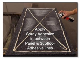
4. Align the panel edges to the side vertical and top horizontal lines, matching the corner of the panel to the corner drawn on the surface. Apply medium pressure on each side to set the edge adhesive, then apply even pressure to the remaining area.
