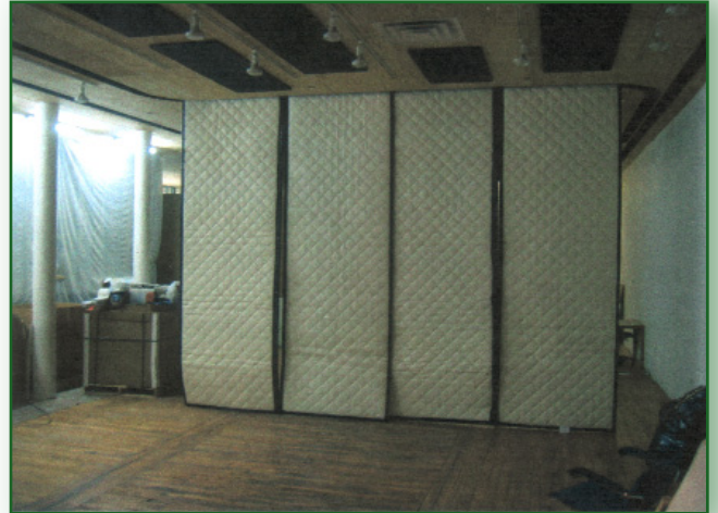
Black Nexxus Studio under construction.
