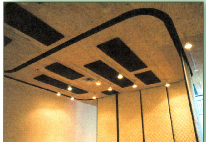
Charcoal Acoustical Surfaces Inc. Sound Silencer Panels P.E.P.P™. overhead help not only with the unique look of the space, but add to the absorption of the room.
