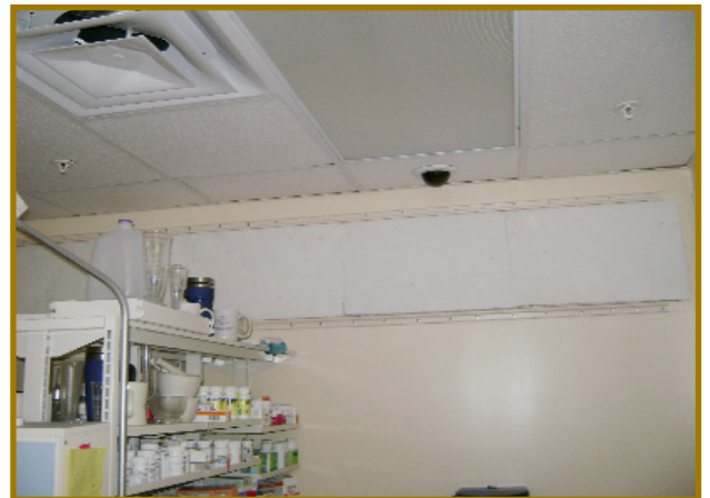
These pictures also show the white Echo Eliminator panels before the fabric was put into place. This installer used button-head screws to hold the WallMate base track to the wall. The picture below shows one long panel that was site fabricated to fit into the room which looks much cleaner than multiple smaller panels installed one next to another.
