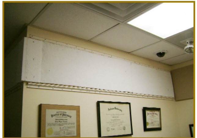
Below: The longer panel shown here shows how the white Echo Eliminator recycled cotton panels are installed onto the existing sheetrock wall before the fabric is stretched over them. The fabric in this system needs to be acoustically invisible so the sound is able to easily pass thru the fabric and be absorbed by the cotton panels.
