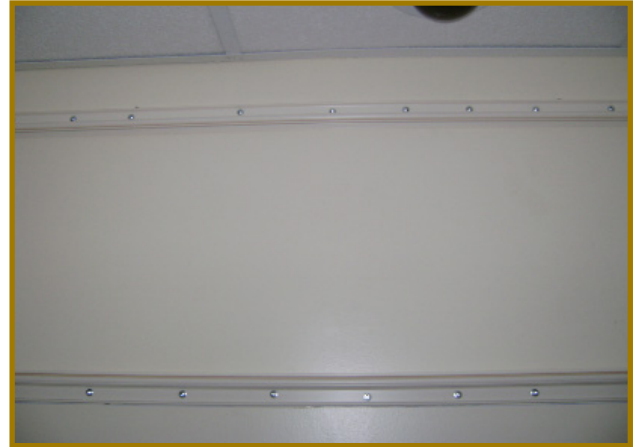
These pictures also show the white Echo Eliminator panels before the fabric was put into place. This installer used button-head screws to hold the WallMate base track to the wall. The picture below shows one long panel that was site fabricated to fit into the room which looks much cleaner than multiple smaller panels installed one next to another.
