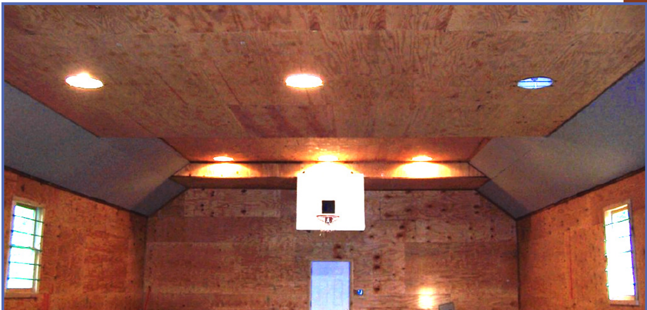
The calculation that I used for the square footage at the Central Advent Church was as follows: The room that they were considering was approximately 40' x 26' x 19' average ceiling height, or approximately 19,760 cubic feet of volume. If I take three-percent of that, I am left with 592.8, which I rounded up and converted into a square footage of panels needed.
