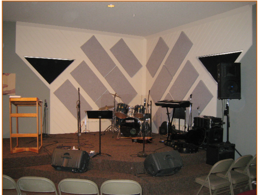
River Heights installed 12 (2' x 4') x 2" thick Echo Eliminator™ panels on the walls behind the stage. Thick panels were two inch. Used to reduce the amount of mid. & low frequencies created by the drums.
