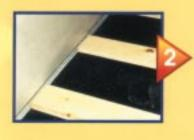
Place the floor furring strips perpendicular to the future floor covering, spaced 12" (305 mm) apart, measured from the center of each strip.
